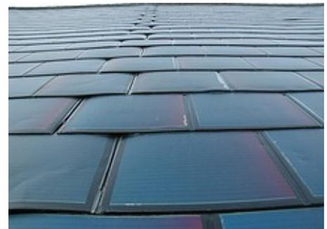
*"triple-junction amorphous silicon thin-film technology incorporated within the Solar Power Tile allows the system to produce an estimated up to 20% more energy than incumbent crystalline silicon panels."*
